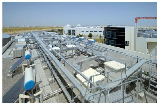
**Image 2 – Solar water heaters & systems in place on roof**
